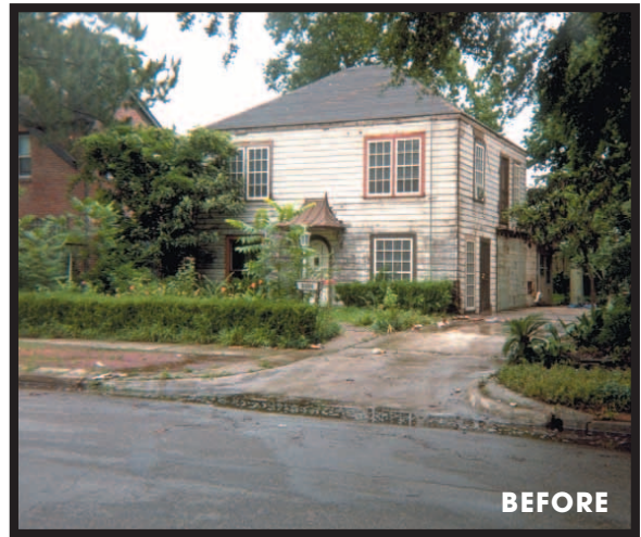
This house in the Rice University area needed major renovation.
